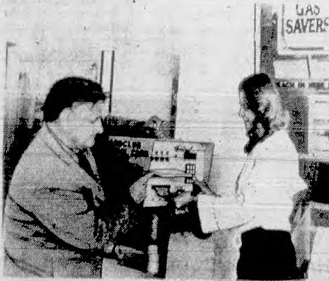
Elmer R. (Woody) Woodard explains the workings of his 1 Rite Time Saver Fuel Control System at his Elizabeth City, N.C., service station. After buying gas and recording her odometer mileage, the customer inserts a credit card into a machine that computes key details of the transaction. Later, she'll get a report on how efficiently she uses fuel.
